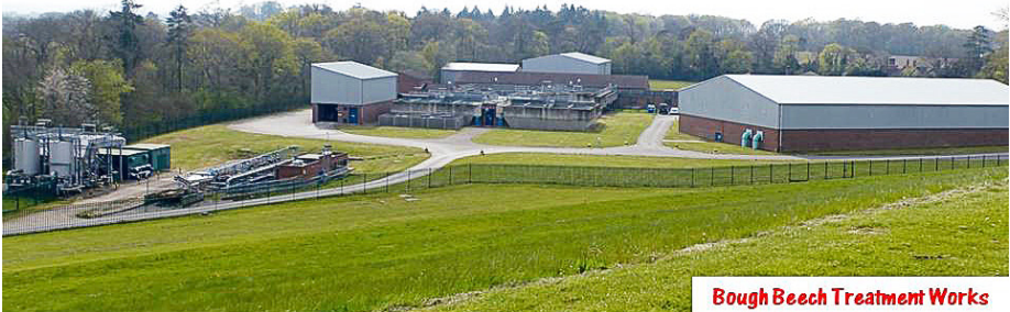
Bough Beech Treatment Works
