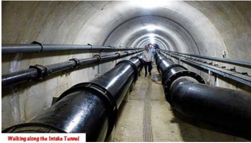
Walking along the Intake Tunnel
